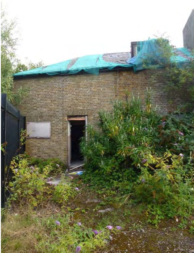
Western cottage facing courtyard
