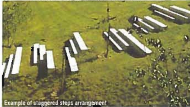
Staggered flights of timber steps to the top of the mound
