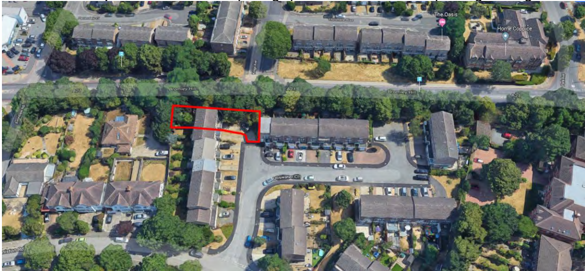
Fig 1. Aerial photograph indicating No.17 Ullswater Close.
